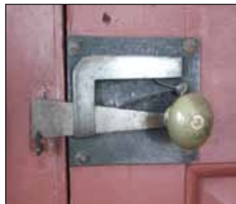
Original 18th-century spring latch on closet door in Dining Room
